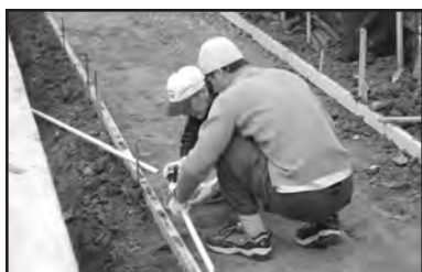
Sally Remedios and her son Matt measure piping.
