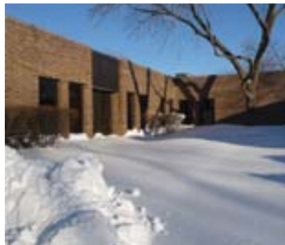
Notice that the door is half covered in snow.
