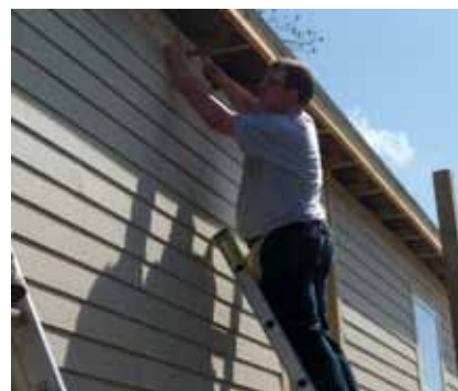
Oliver Schottke hammers in the last of the siding
