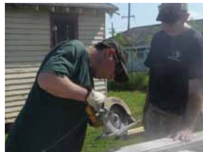
C.J. Lagan and Jack Krecek work the saw
