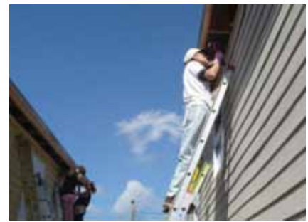
Sally Remedios works on residing the house
