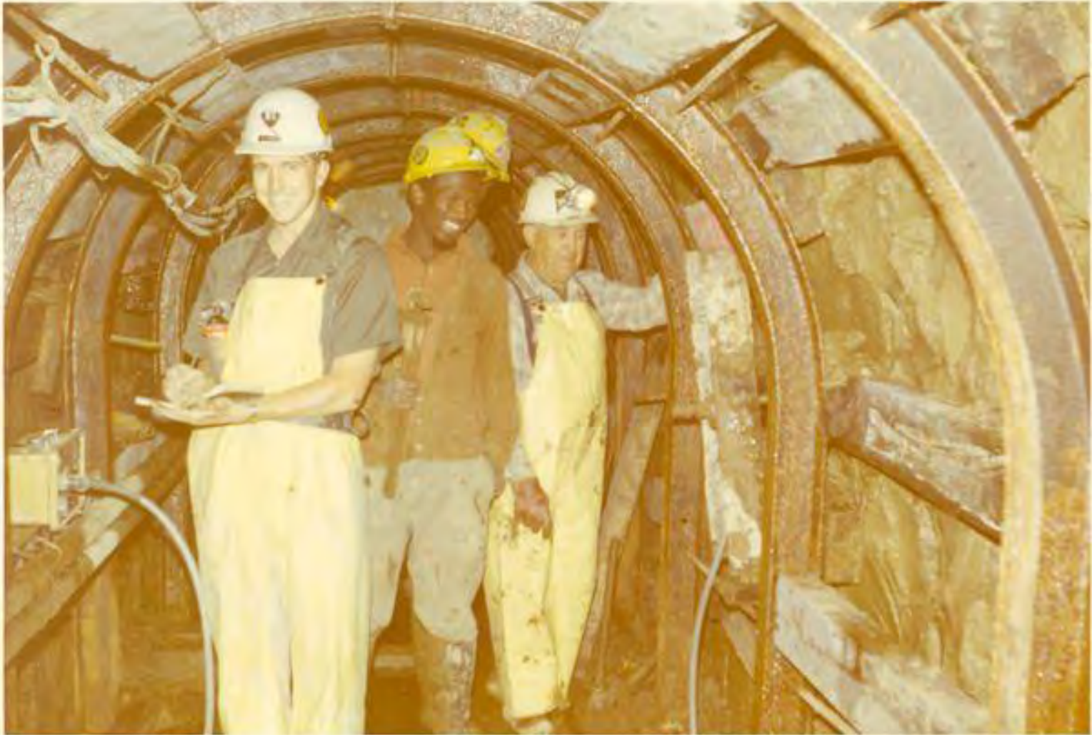
Sewer tunnel system construction, c. 1969.
