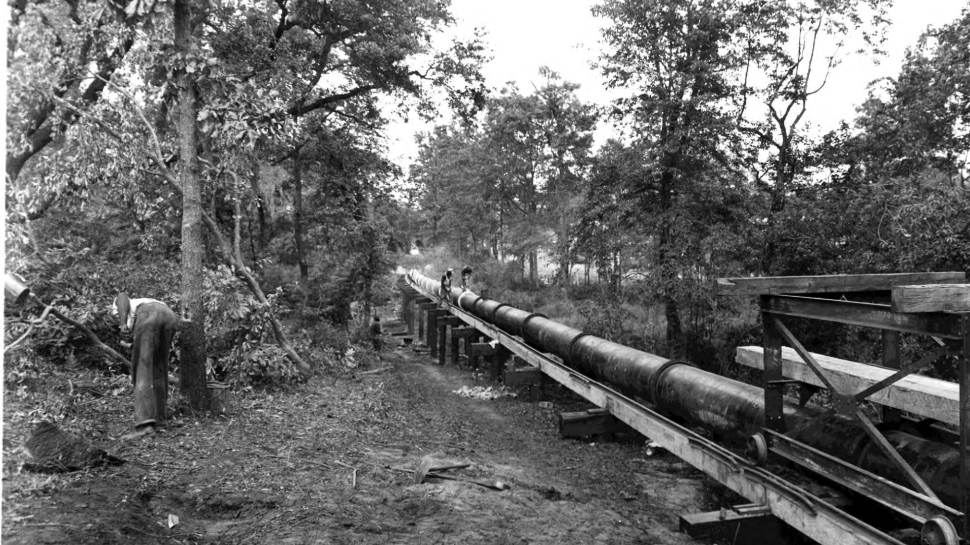
TRESTLE & PIPE COMPLETED. TAKING UP TRACK, WEST TRESTLE, NOISETTE CR. AT RHETT & HELM AVE'S. AUG. 13. 1941.
