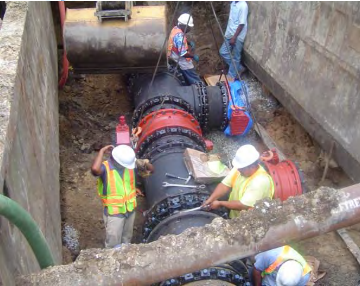
30-inch water main, Grimball Road, James Island, Winter 2007.
