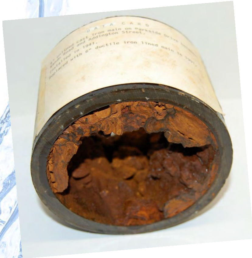
Cross section of cast iron water main, cir. 1941, replaced 1991.
