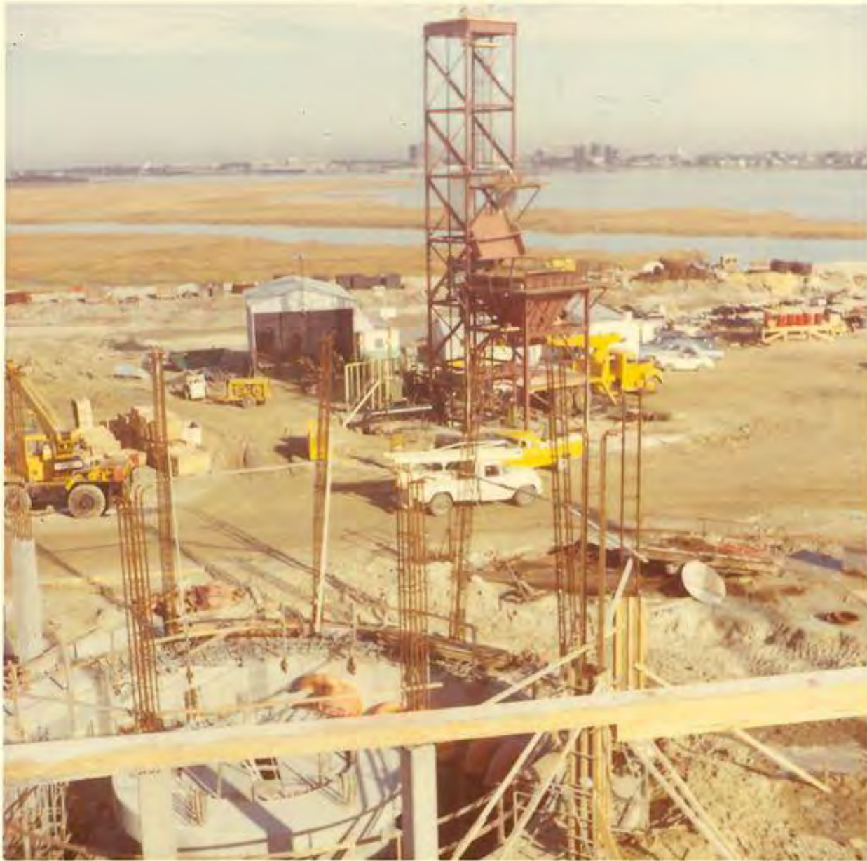
Plum Island Wastewater Treatment Plant construction, c. 1969.
